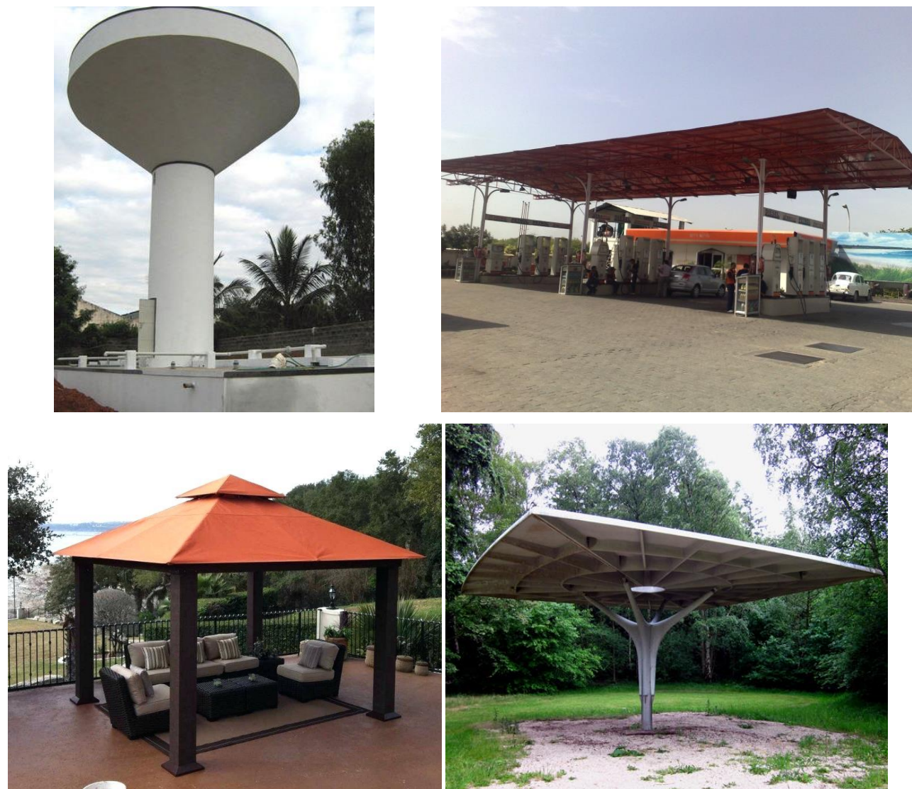
Figure 2-1: Some examples of structures which can be idealized as a single-degree-of-freedom (SDF) systems
