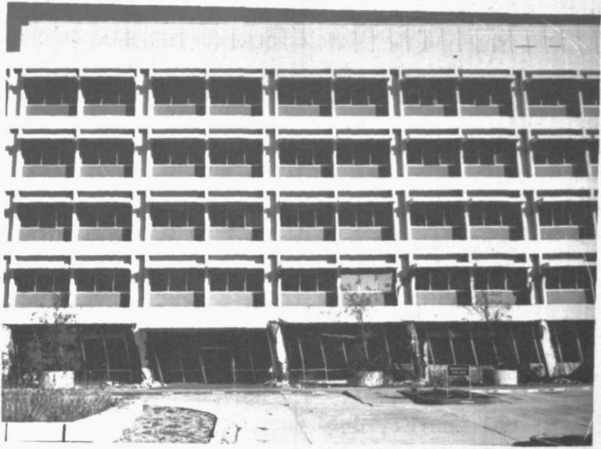
Olive View Hospital after February 1971 San Fernando earthquake
