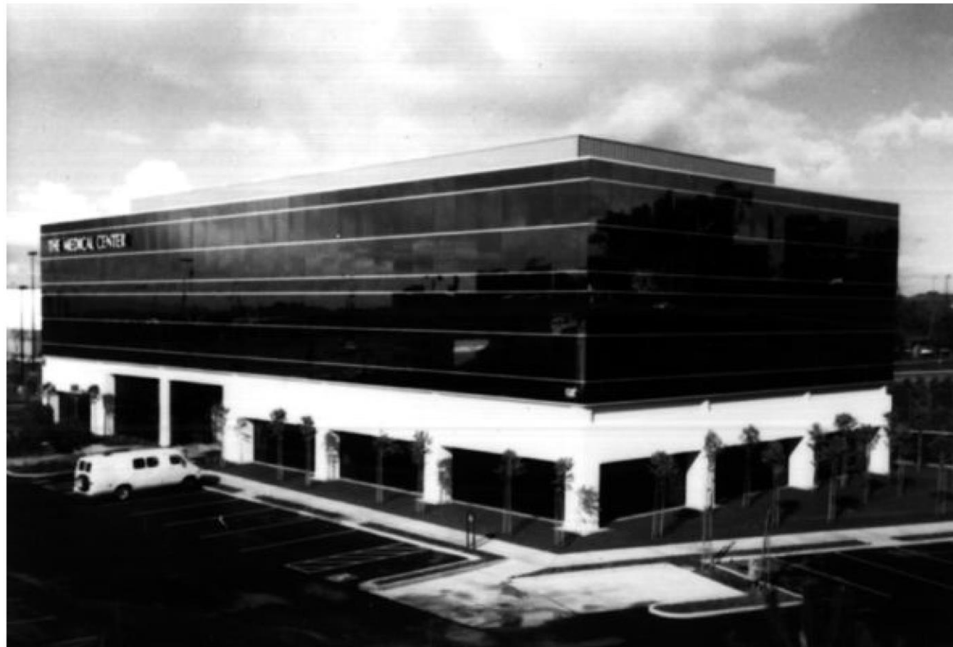
Figure 2.1.2c Medical Center Building, Richmond, California. The fundamental natural vibration periods of this three-story steel frame building are 0.63 sec for vibration in the long direction, 0.74 sec in the short direction, and 0.46 sec for torsional vibration about a vertical axis. These vibration properties were determined from motions of the building recorded during the 1989 Loma Prieta earthquake. (Courtesy of California Strong Motion Instrumentation Program.)
