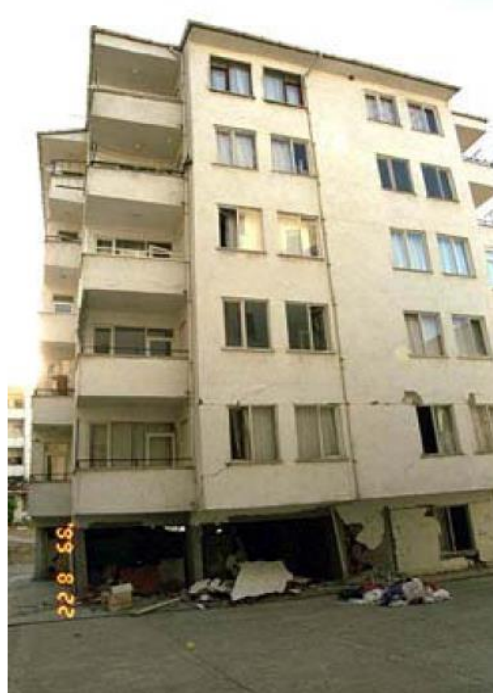
Infill-Failure Induced Soft/Weak Story
