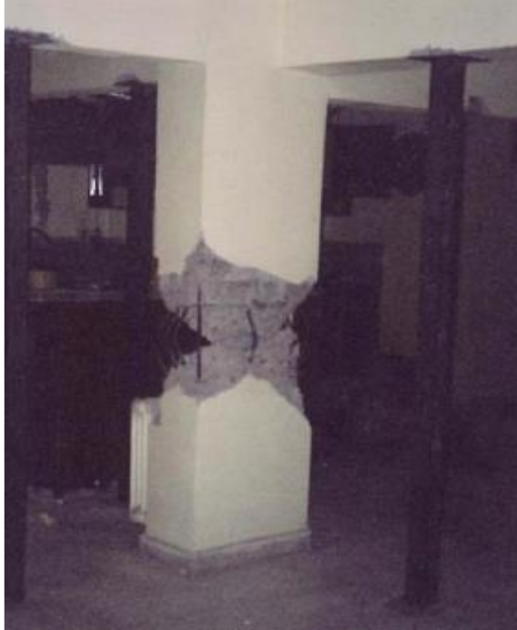
Lap-Splice Failure in Columns
