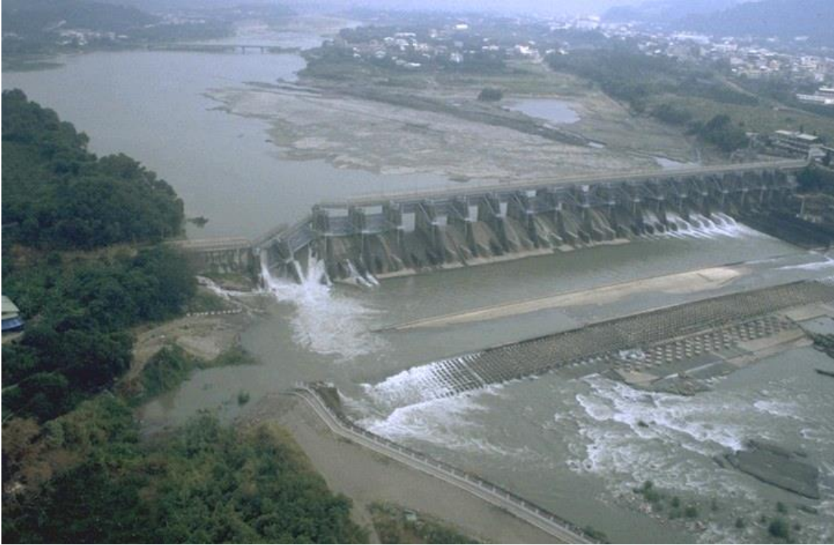
Surface Rupture Hazard: The 1999 Chi-Chi earthquake, Taiwan
