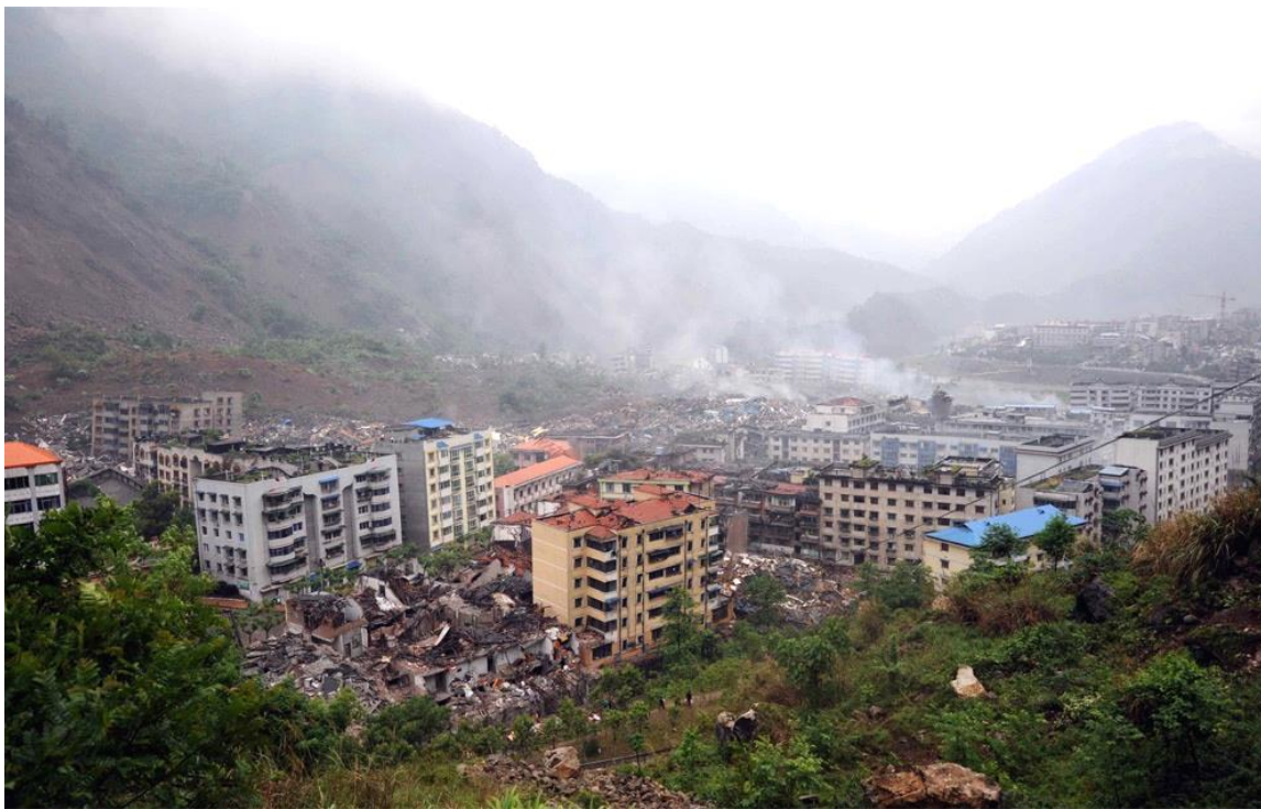
Ground Shaking Hazard: Wenchuan Earthquake (2008), China ( Magnitude = 8.0 )
