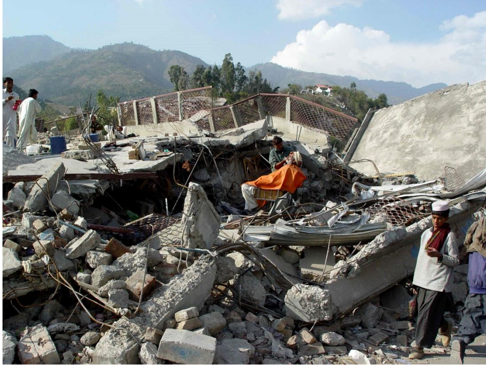
Ground Shaking Hazard: Kashmir Earthquake (2005), Balakot, Pakistan ( Magnitude = 7.7 )
